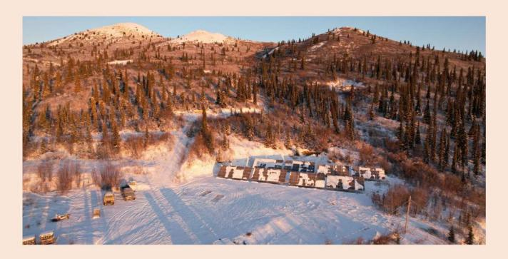
Two arrays of solar panels were installed on site in October 2023: one at the Water Treatment Plant and one at the bunkhouse. The solar panels will reduce the use of generators, fuel consumption, and CO2 emissions at the site, notably in the summer when daylight hours are long.
